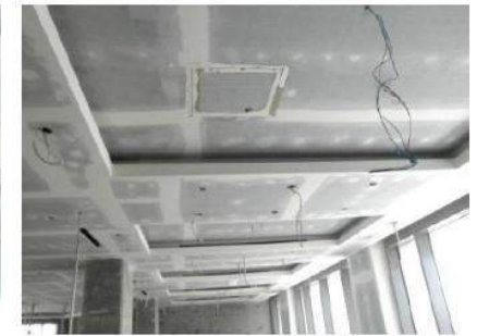
Two Level Gypsum Ceiling
