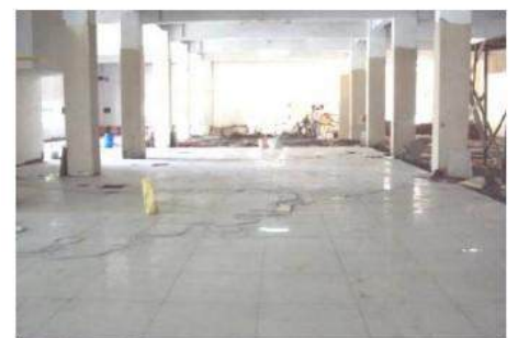
Tiles Fixing, Flooring
