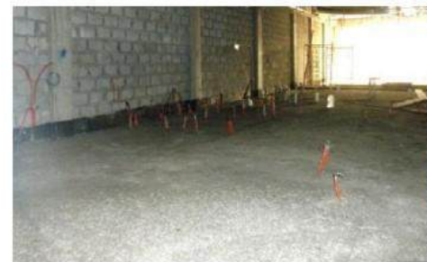
Interior Civil Work, Screed
