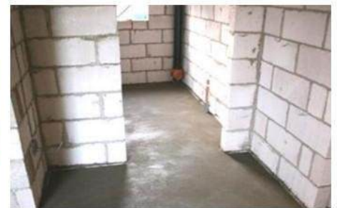
Interior Civil Work, Block
