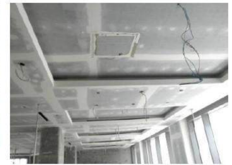
Two Level Gypsum Ceiling
