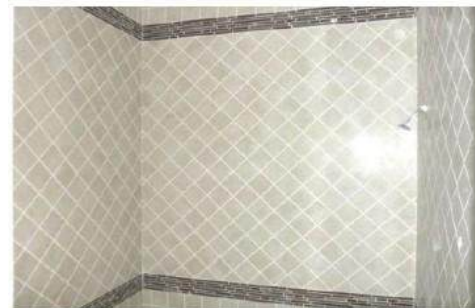
Tiles Fixing, Wall Tiles
