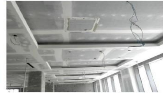
Two Level Gypsum Ceiling
