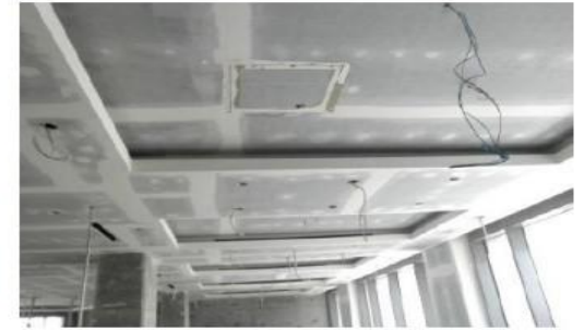
Two Level Gypsum Ceiling
